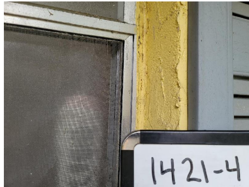
1421-4 Caulk Typical Exterior Windows
